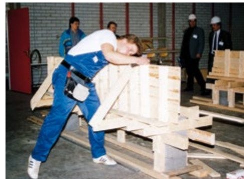
In the construction industry competition, the competitors built a wooden mould for a reinforced concrete beam on the first day, and reinforced the beam and its projection on the second day.
